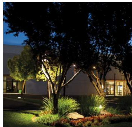
Tree downlights - "Moonlighting"
