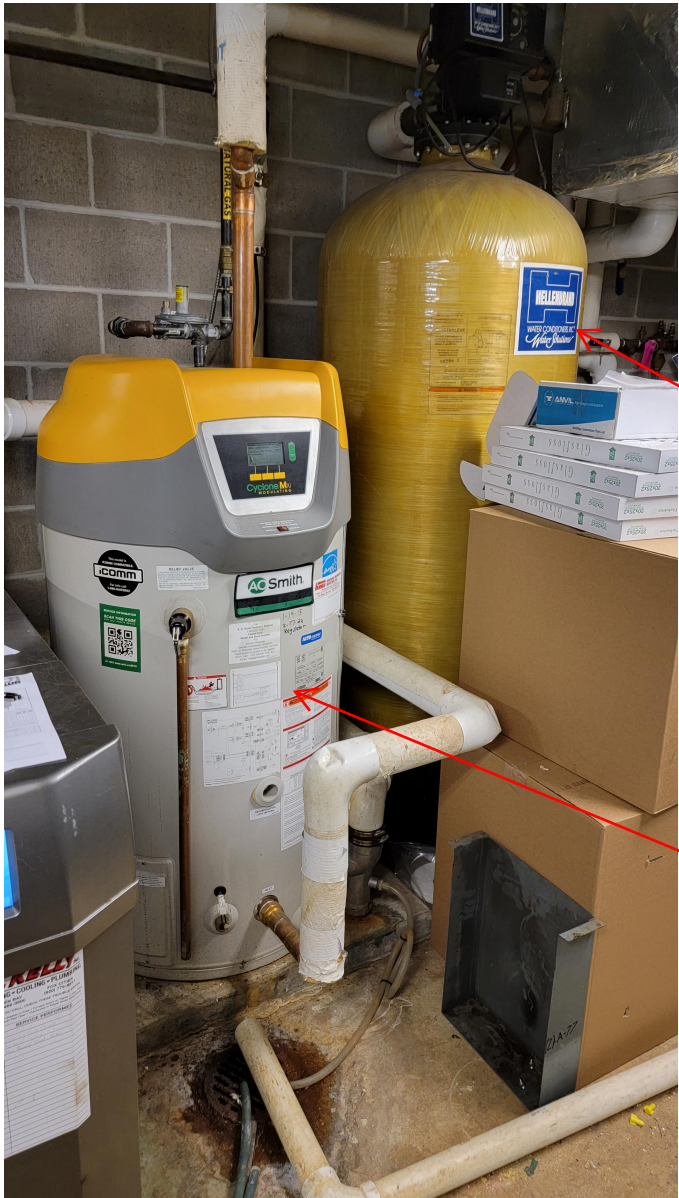
WATER HEATER & WATER SOFTENER
