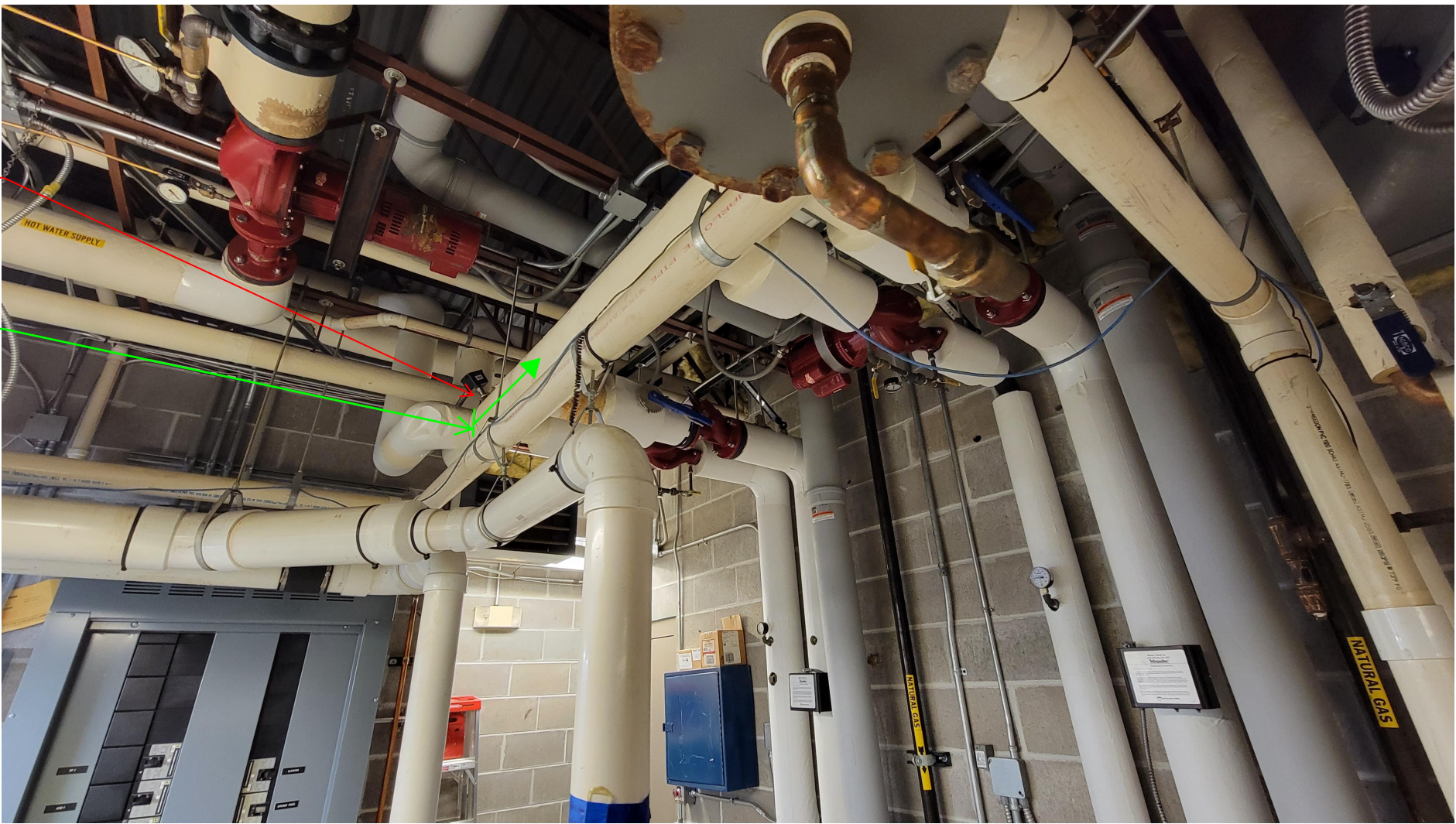
REMOVE & REINSTALL HOT WATER SENSOR IN SECONDARY PIPING
