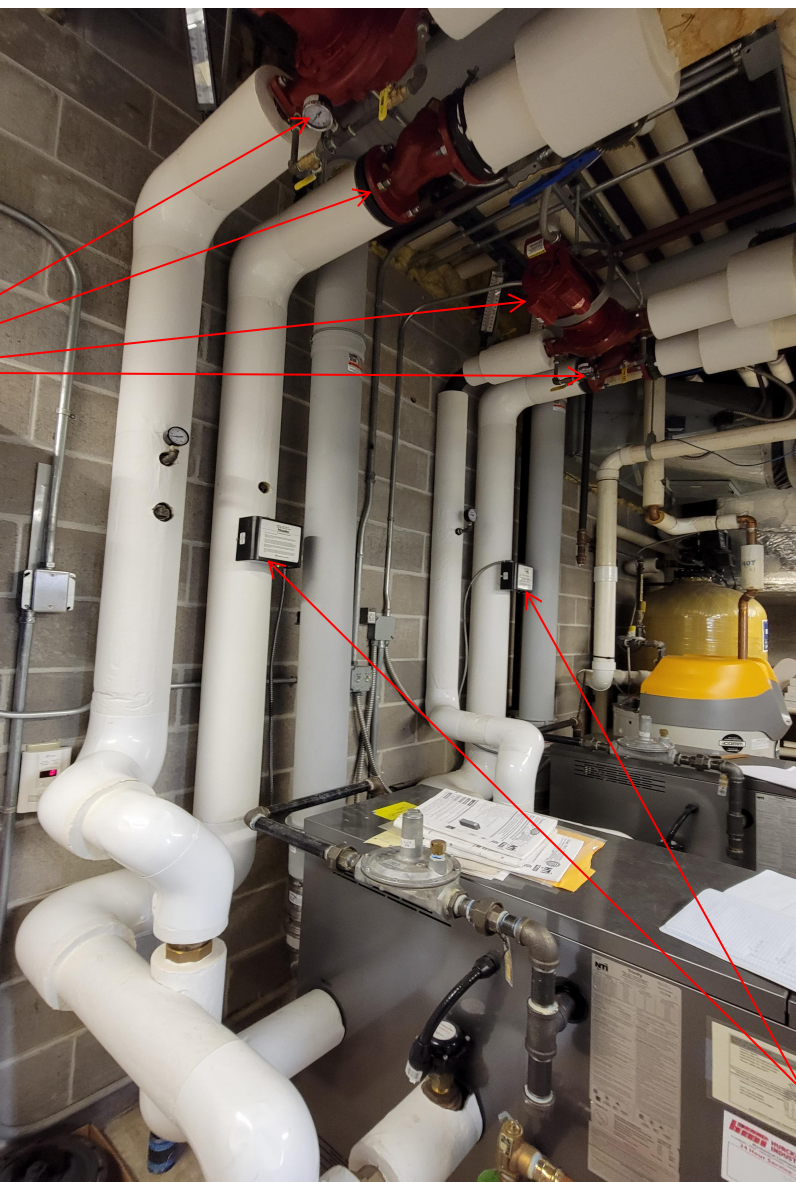
BOILER PIPING PUMPS, TRIPLE DUTY VALVES
