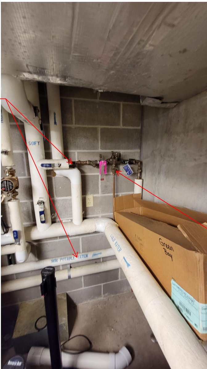
RELOCATE TESTABLE RPZ VALVE
