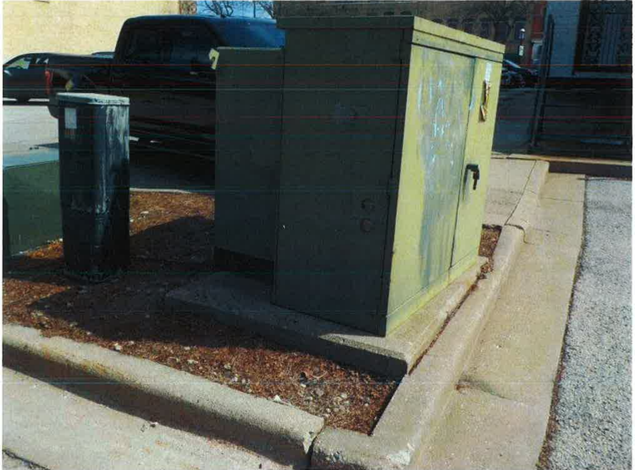
Pad mounted transformer along south property line.
