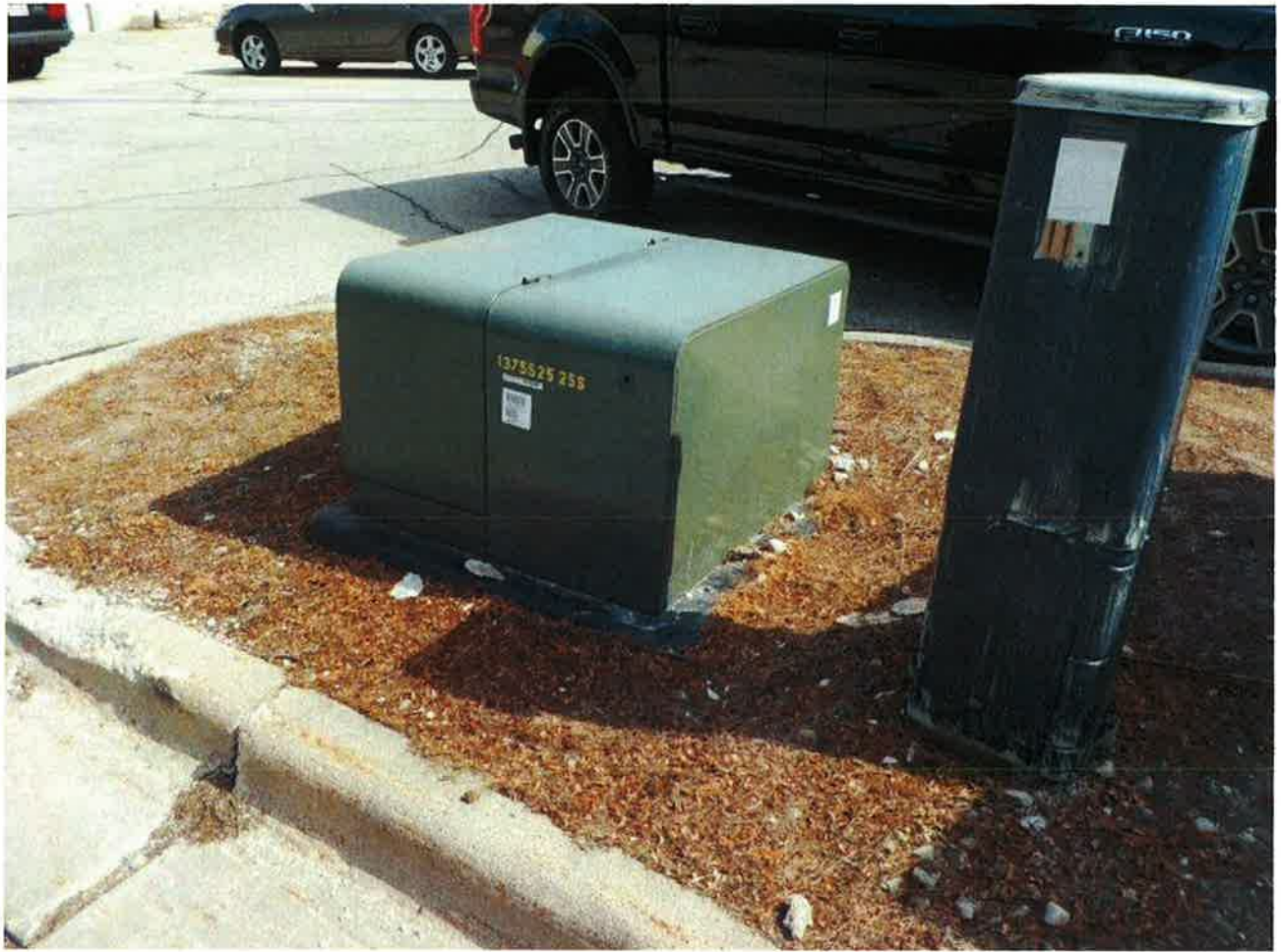
Pad mounted transformer along south property line.
