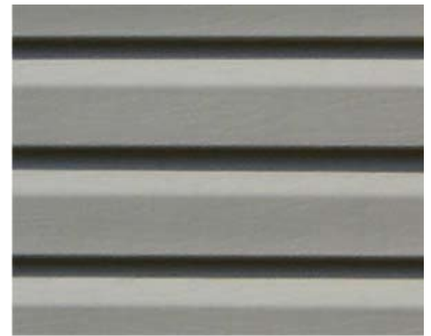
Top: Good example of vinyl siding.
