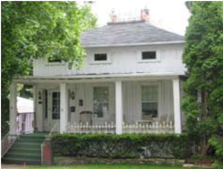
410 Fulton St. Greek Revival
