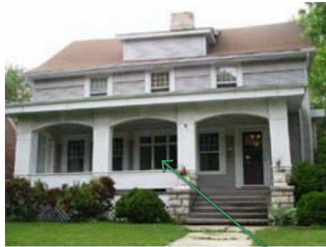
449 N. Wisconsin St. Colonial Revival
