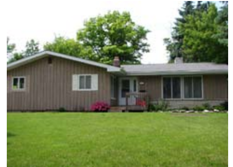
953 Oakdale Ave. Contemporary
