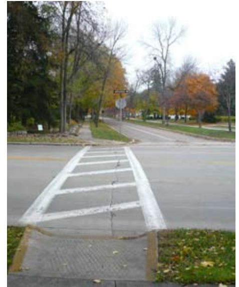
Crossing at Broadway and Ridgeway Boulevard
