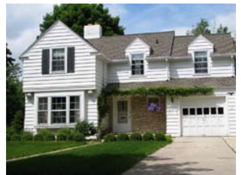
703 Ridgeway Blvd. Gable Ell
