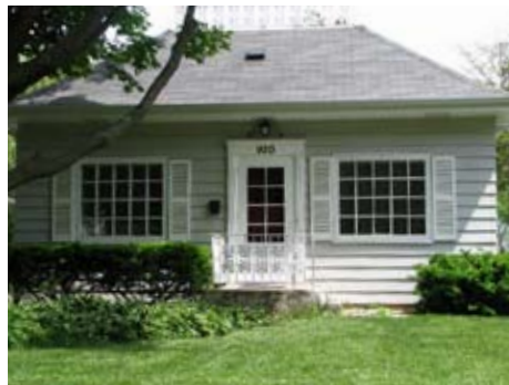
920 Oakdale Ave. One-story Cube
