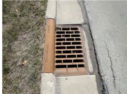
...but perpendicular grates allow bikers to cross them safely.
