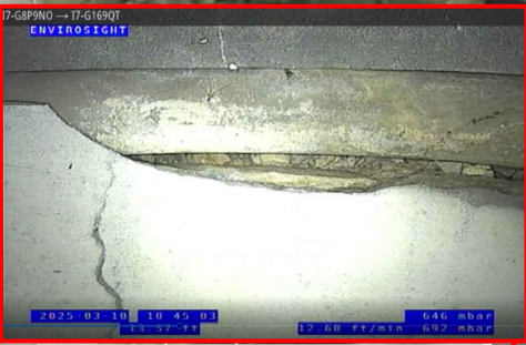
TV OF SEPARATED JOINT 10' EAST OF STMH
