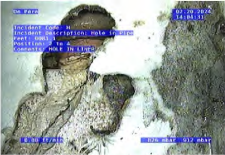
H - Hole in Pipe @ 81.1 ft. HOLE IN LINER
