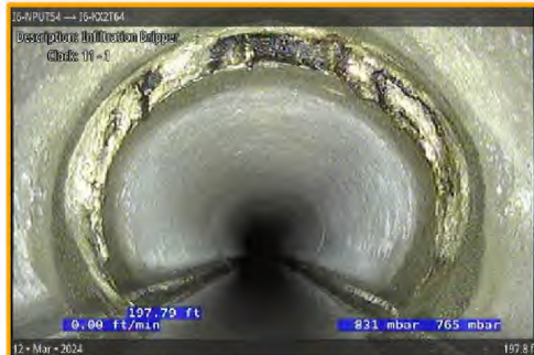
[Grade 3] Infiltration Drinker at 197.8 ft, 11 - 1 o'clock
