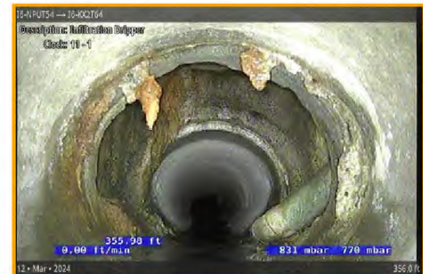
[Grade 3] Infiltration Drinker at 356.0 ft, 11 - 1 o'clock
