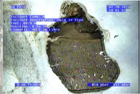
H - Hole in Pipe @ 79.0 ft. HOLE IN LINER
