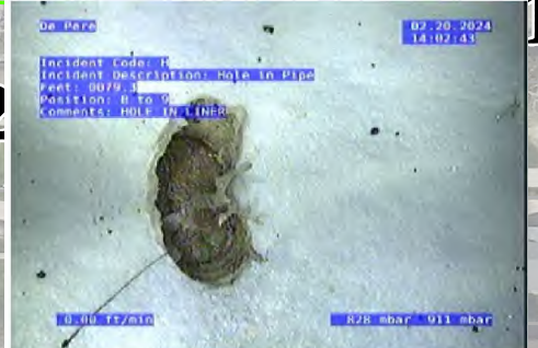
H - Hole in Pipe @ 79.3 ft. HOLE IN LINER
