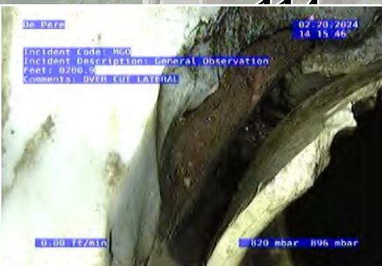
MGO - General Observation @ 200.9 ft. OVER CUT LATERAL
