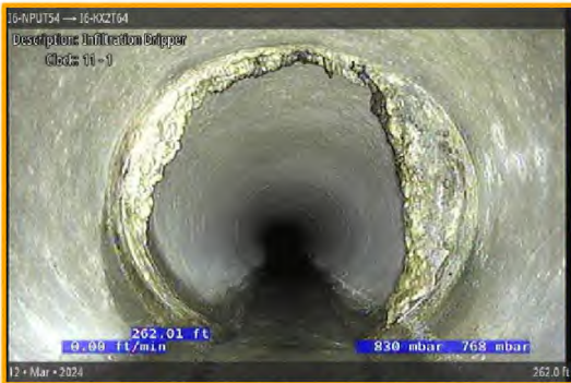
[Grade 3] Infiltration Drinker at 262.0 ft, 11 - 1 o'clock
