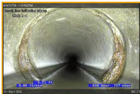
[Grade 3] Infiltration Drinker at 005.7 ft, 2 - 4 o'clock
