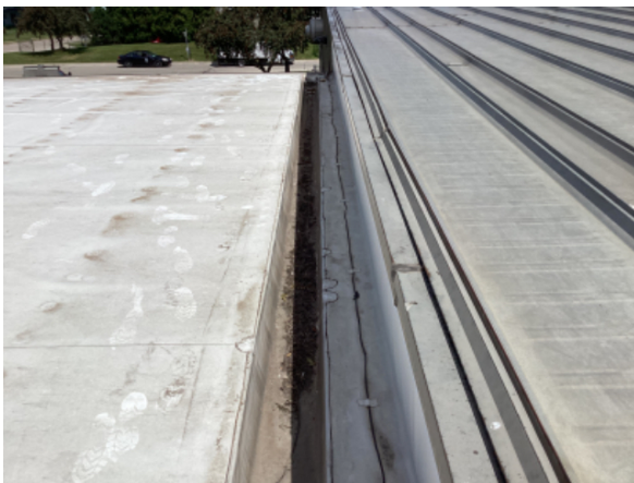
Internal gutter flashing on non leaking portion of the roof.
