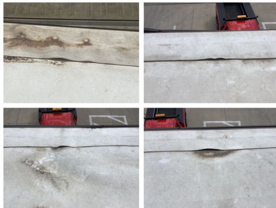
Leaking edge strip at gutter is typical
