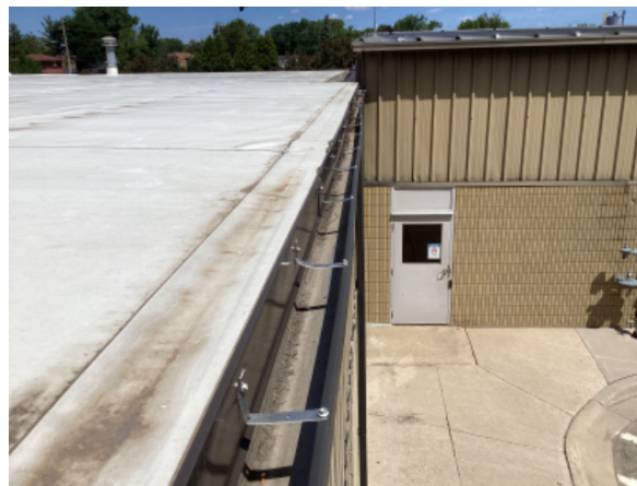
Gutter rests on shelf flashing
