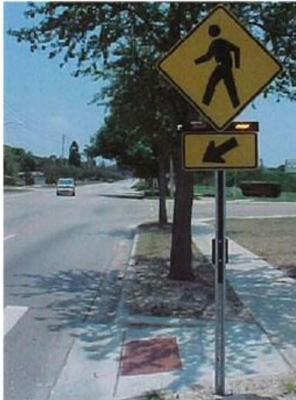
RRFB's can enhance pedestrian safety by reducing crashes between vehicles and pedestrians at unsignalized intersections and mid-block pedestrian crossings. According Federal Highway Administration (FHWA) research, installing RRFB's at a marked crosswalk can increase driver yielding to pedestrian patterns to between 80% and 100%.
